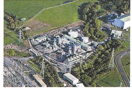
Powering up: Contact Energy's Stratford Power Stations. The new Stratford Peaker Plant is to the left of the older Taranaki Combined Cycle station, at the rear of the site.
